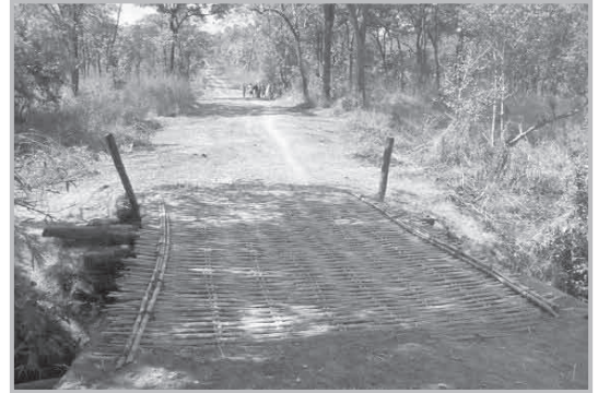
Bridge made of bamboo in Mozambique
