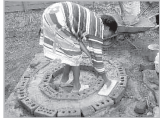
Making a concrete ring beam
