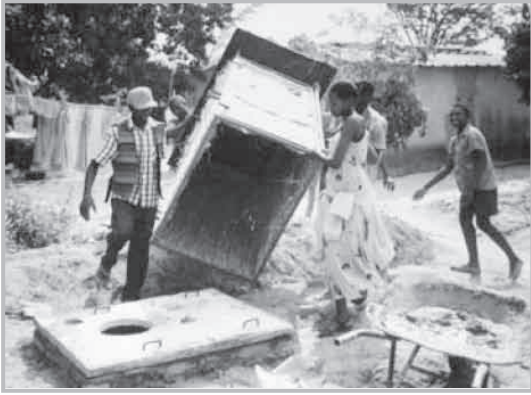
Placing a movable structure.
