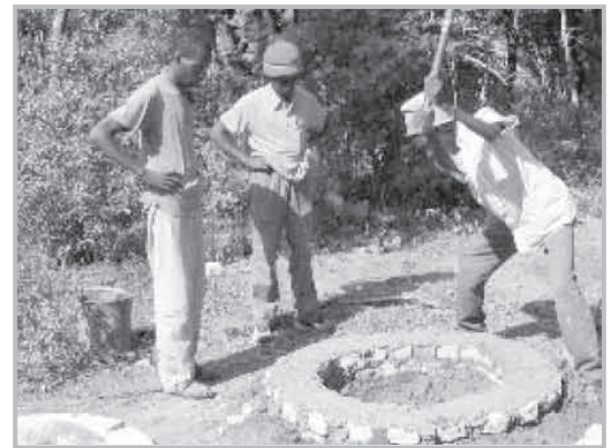
Digging inside the ring beam
