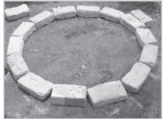
Mould for a slab. Placing the plastic
